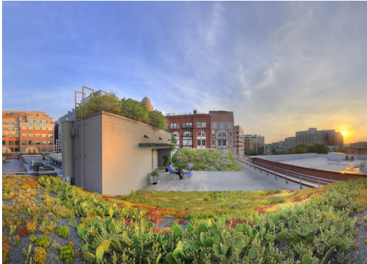
American Society of Landscape Architects Headquarters, Washington DC
