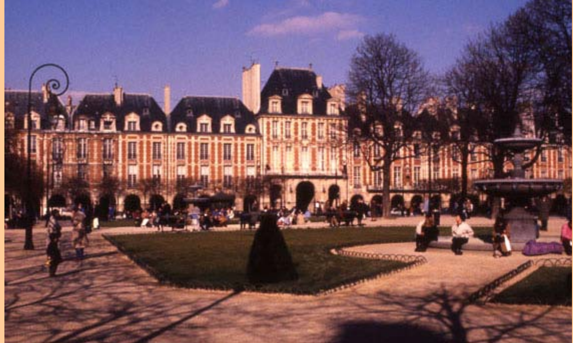
Protection of the urban grain in the historic core Place des Vosges, Marais quarter
