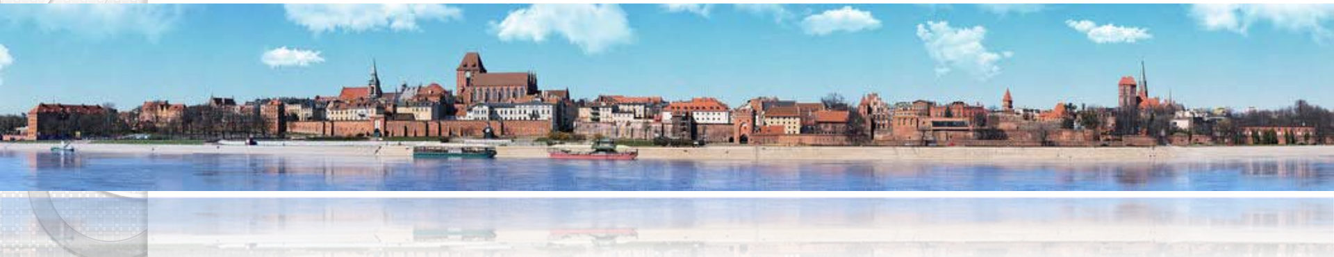
The chain of the medieval defence walls along the Vistula River, restored 2010-2012
