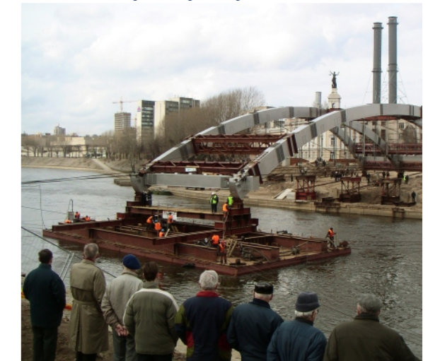
Karaliaus Mindaugo tilto statyba Construction of King Mindaugas bridge
